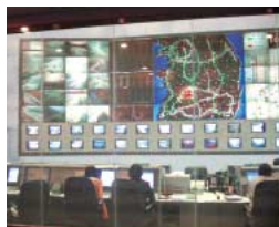
Traffic control center
